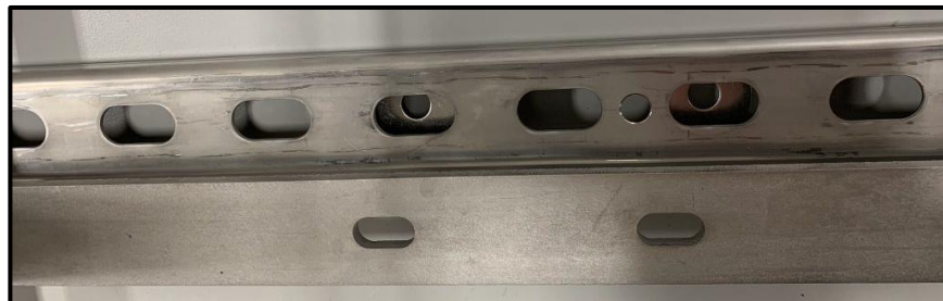
Figure 13: Top view of alignment for hex cap bolt installation.
